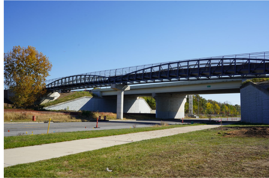
Pedestrian Bridge along CR 17 over US 33
